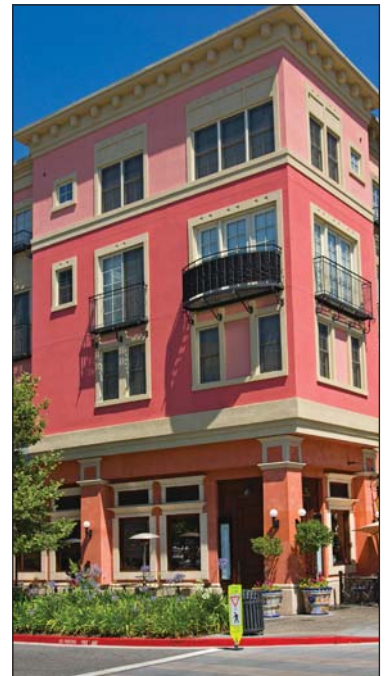
Example of 3-4 storey residential buildings
