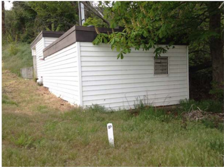
West Kelowna Estates Intake Pump Station
