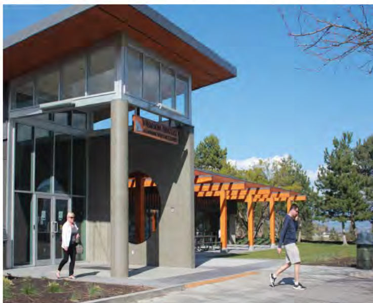
New foyer and pergola at JBMAC.
