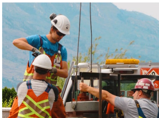
Figure 16: Crews performing maintenance work
