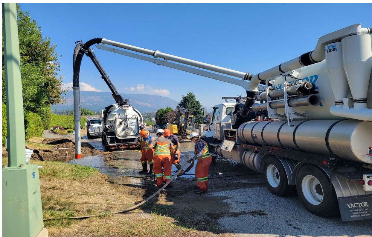
Figure 15: Crews fixing a water main break in West Kelowna
