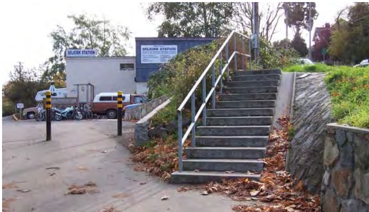
Figure 28: Stairway with Bicycle Wheeling Channel in Victoria West
