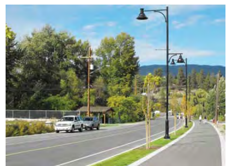
Phase 1 Gellatly Streetscape Enhancements
