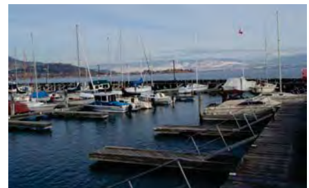
Existing moorage at the WKYC.
