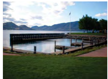
Day moorage with breakwater in Peachland
