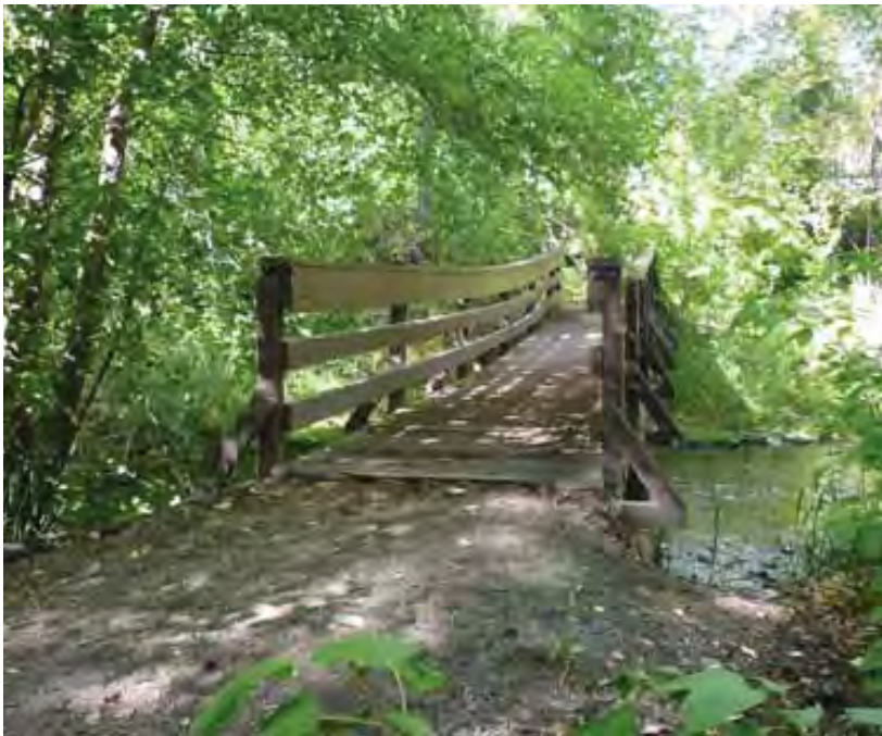
Pedestrian bridge over Powers Creek
