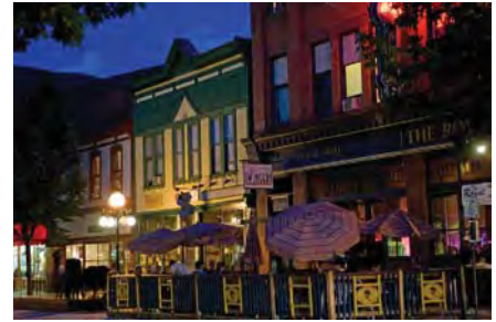
Nelson, BC has capitalized on its historic buildings, with thriving commercial frontages and office and residential above.
