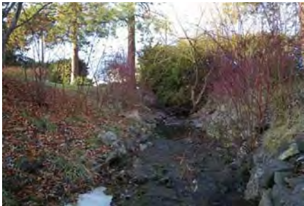
Rip rap shoreline on McDougall Creek
