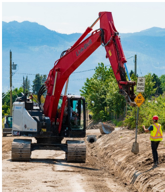
Figure 5: Crews working on the Menu Road Upgrades
