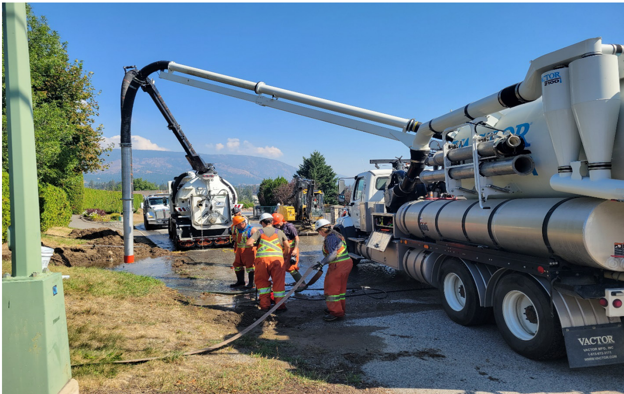
Figure 14: Crews fixing a water main break in West Kelowna
