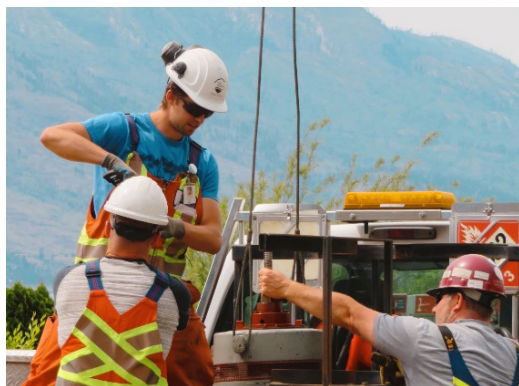
Figure 15: Crews performing maintenance work
