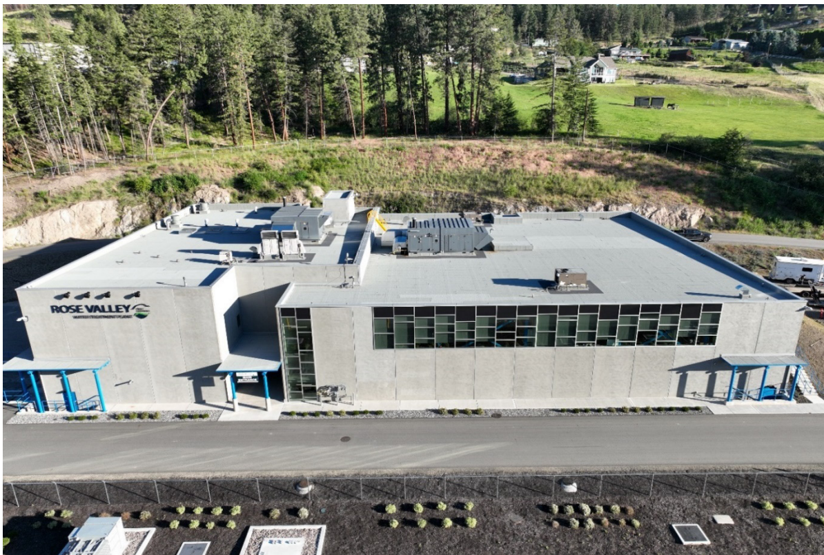
Figure 7: Rose Valley Water Treatment Plant
