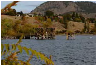
CNR Wharf from the water
