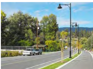
Completed Gellatly Road and corridor upgrades between the Cove Resort and Kent Park
