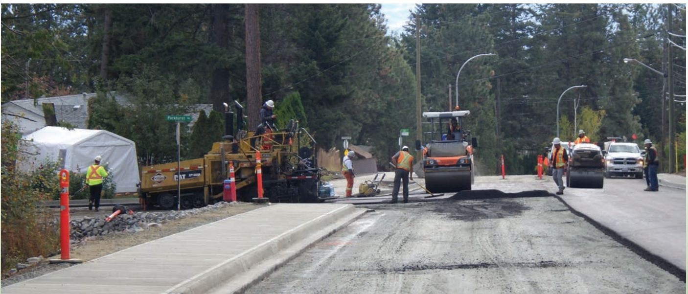
Glenrosa Road construction
