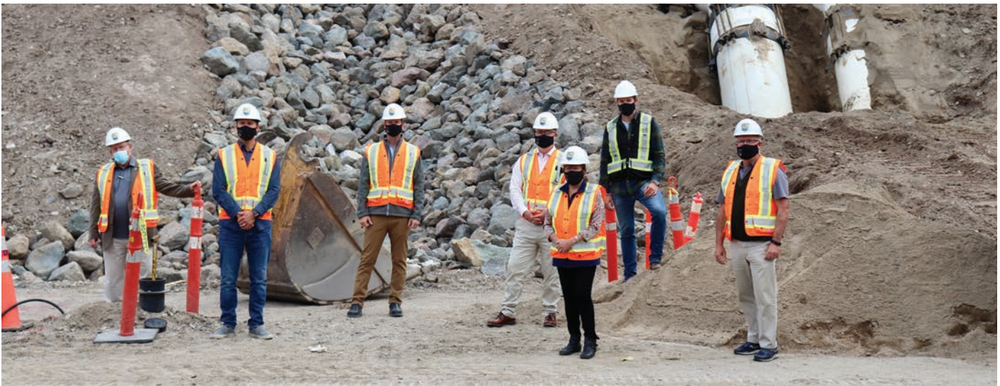
Council's site visit of Rose Valley Water Treatment Plant construction
