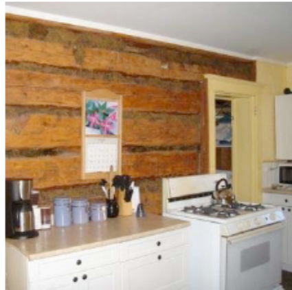
Photo 2: Kitchen showing original logs and chinking
