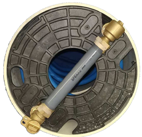
Top view of a typical water meter pit purchased and installed by owner.
